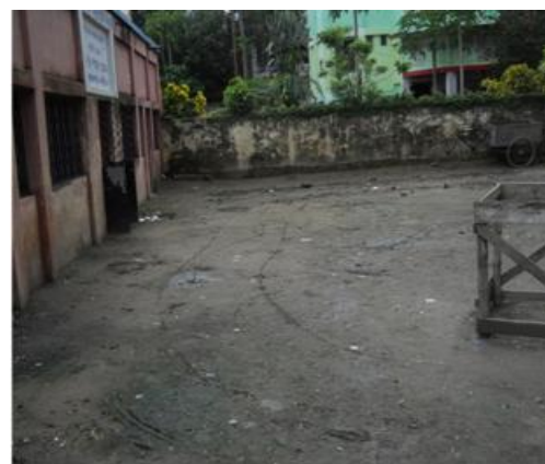
Plate 4: Poor Play ground Structure of Nicer Para Primary School, Krishnagar
