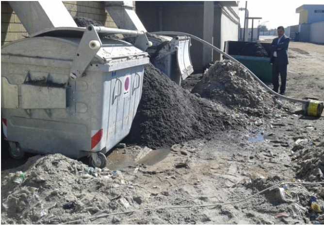
Photo 1: Heavy production of grits from aerated grit chamber of 50,000 m 3 /day capacity new municipal wastewater treatment plant of Kufa, Iraq
