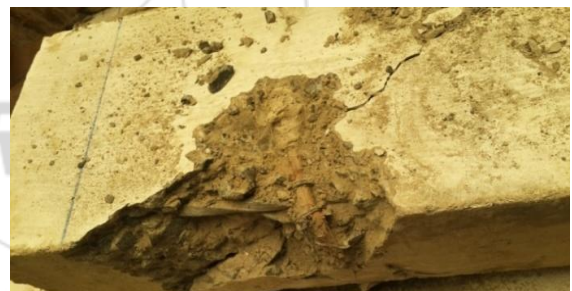
Fig.10: Unbroken shear reinforcement for L.B.1x8 beam
