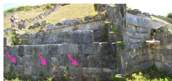
Figure 17: a) frontal view of the basin wall [5] Notice three holes which poured water into the draw basin. b) lateral overflow of the first basin.[5]
