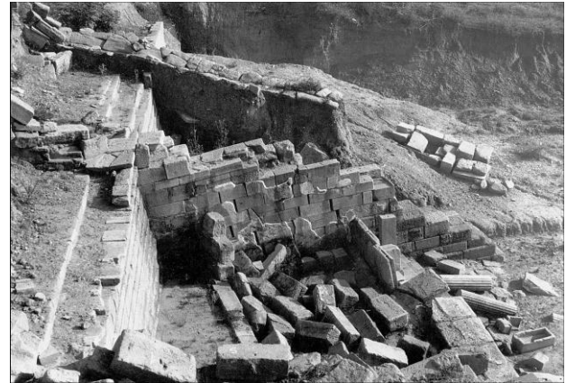
Figure 16: Aerial view of Apollonia fountain while discovered, prior the anastylosis proces of 1974. Note the open holes due the shunt of isodomics blocs on the lateral walls of the basins. [23]
