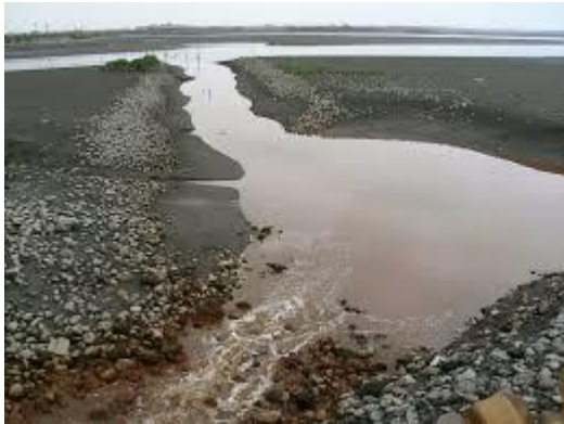
Figure 2: Untreated water being fed into river
