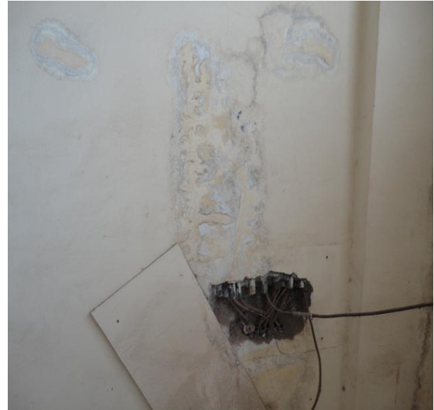
Distress Found in Switch Board
