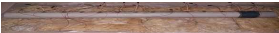
Figure 1.6: Photographic view of preparing for packing/rapping the Glass Wool (insulation) over the 1.6m long pipe for proper insulation
