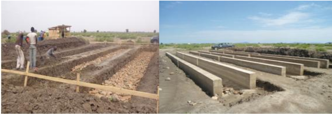
Figure 8: Foundation for the implementation of the solar panels
