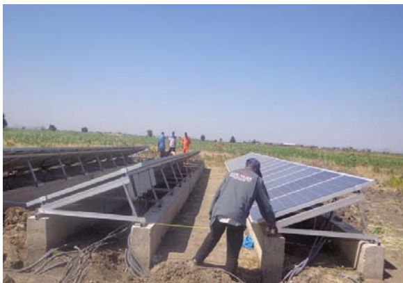
Figure 9a: Fixation of PV panel cables
