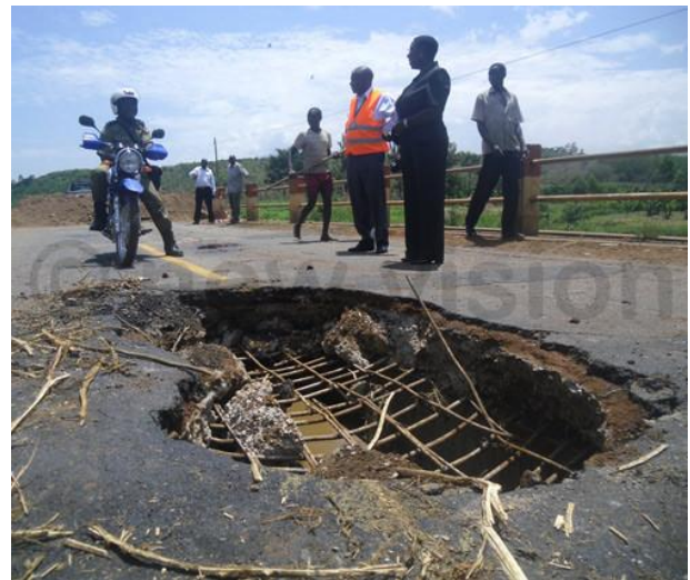
Figure 1: Cracks in the Manafa bridge (The slab may not have been connected to the steel girder using studs)
