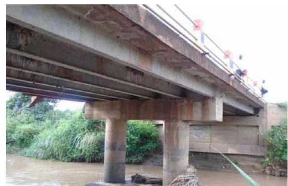
Figure 5: Bridge underside showing steel beams and pier.
