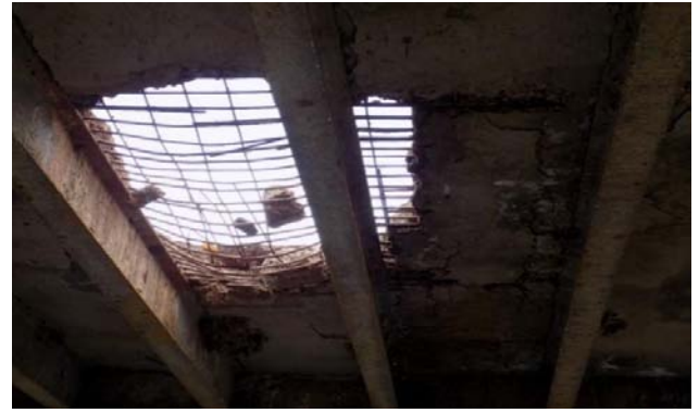
Figure 10: Opening in superstructure slab as seen from underneath the Bridge
