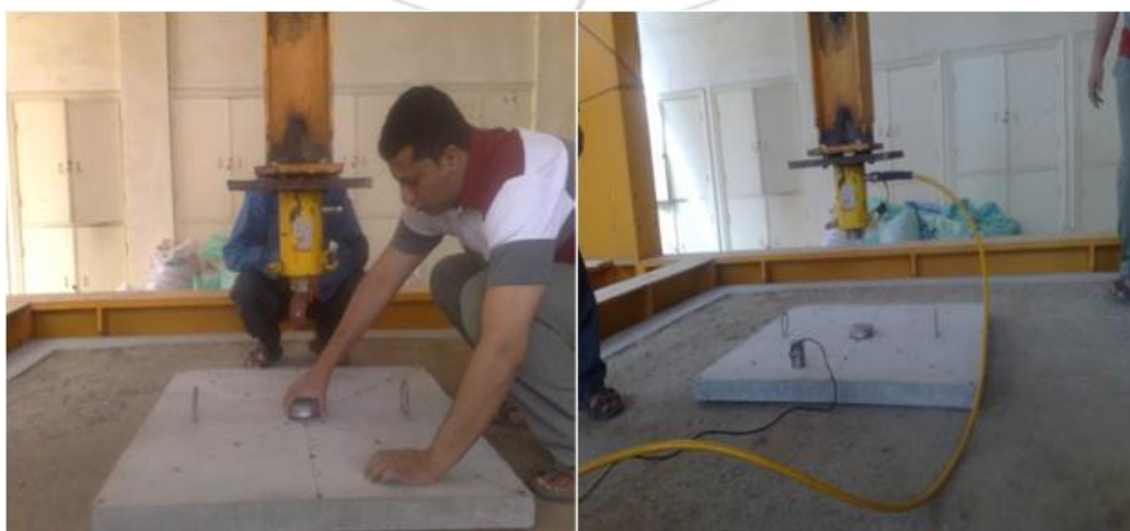
Photo 2: Test of slabs
