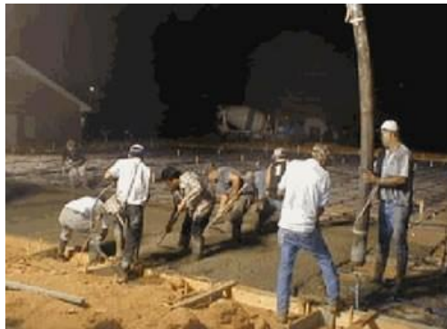
Figure 2: Pouring of concrete in Night
