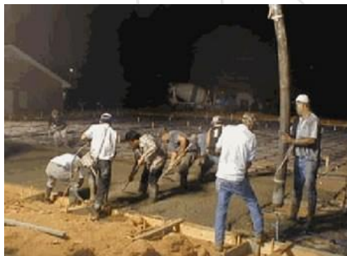
Figure 2: Pouring of concrete in Night
