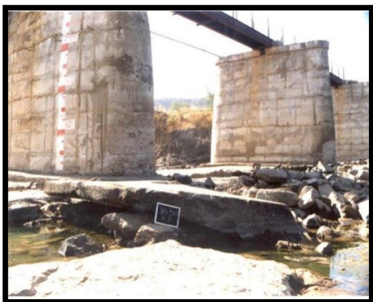
Figure 8: Scouring on Hard Rock
