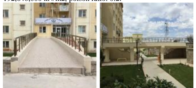
Figure 4.1.1: Front view Figure 4.1.2: Side view Figure 4.1: Views of the SPU Footbridge
