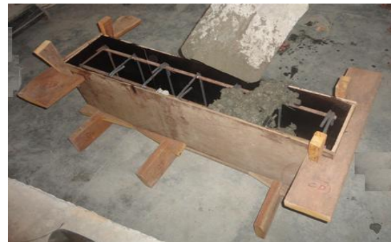
Figure 2: Casting of Control Beam
