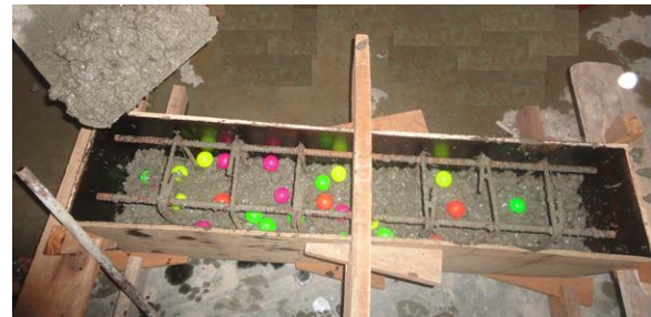
Figure 3: Casting of Replaced Beam
