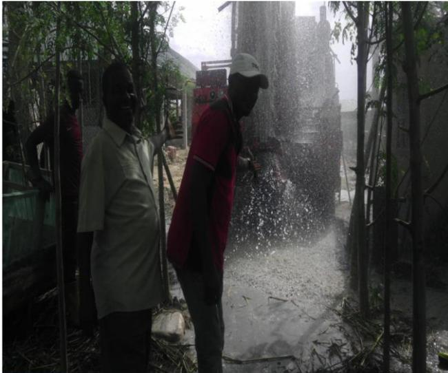
**Plate 3:** Substantial amount of water during drilling of borehole at VES2 station which was one of the two points that were recommended for drilling
