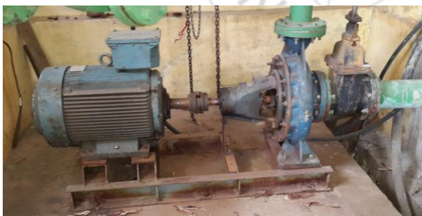
Figure 1: Centrifugal Pump Set-up [BHEL Bhopal Source]
