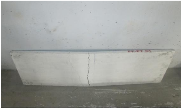
Figure 11: (a) Crack Pattern (FP-FT01)
