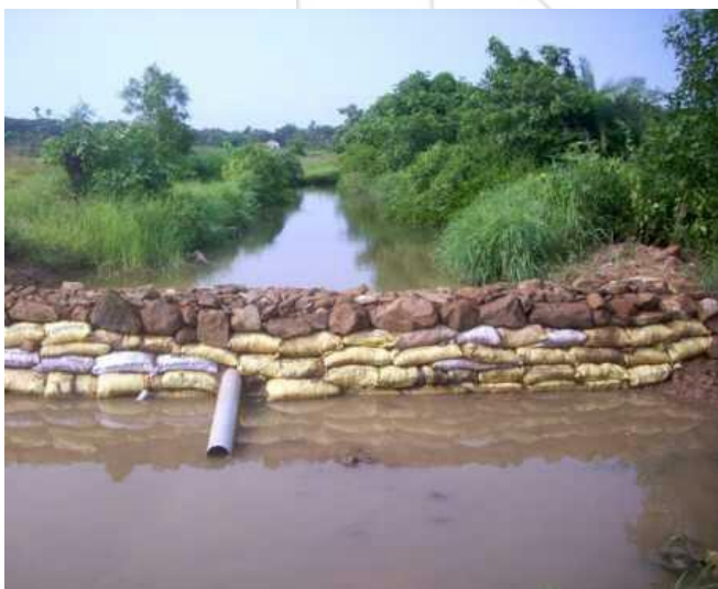
Photo No.3: construction of Vanrai bandhara
