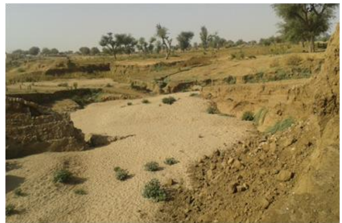
Figure 5: Sediment deposition in the reservoir area
