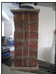
Figure 5: Vertical Splitting Cracks
