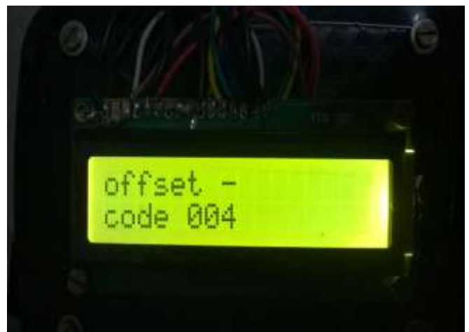
Figure 6(b): LED display showing Offset Misalignment
