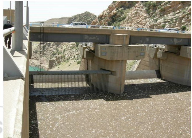
Figure 2: Spillway gate No. 3 of Darbandikhan Dam.
