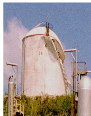
a) Elephant-foot buckling b) Damage to the roof or the Upper shell of the tank
