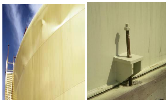
c) Sloshing damage to the d) Inelastic stretching of an upper shell of the tank anchor bolt at the tank base
