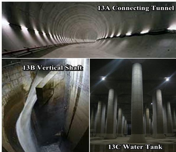
Figure 13: (A) Connecting Tunnel, (B) Vertical Shaft, (C) Water Tank of MAOUDC (Source: Web Japan, 2012)
