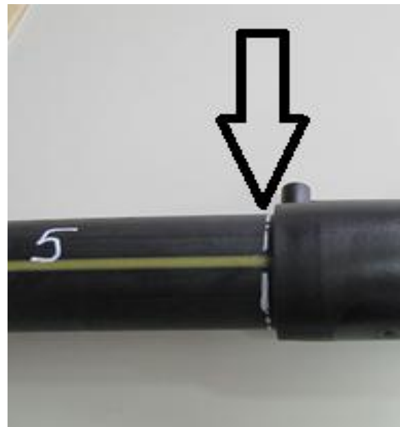
Figure 6: Marking the length of the Dn32 elbow on the pipe
