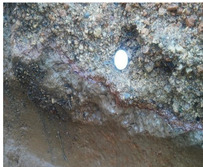
Figure 7: Saturation of sliding surface during and after the rainfall
