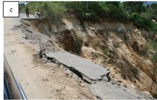
Figure 4: (a) Flowslide showing long travel distance (b) Morphology of landslide around Manggur Gadang River (c) scarp of the landslide with slope with 30° slope
