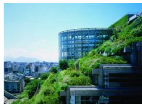
Figure 3.3: The ACROS Building, Fukuoka, Japan is an intensive green roof example
