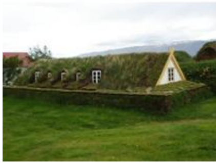
Figure 2: Turf roof – Iceland
