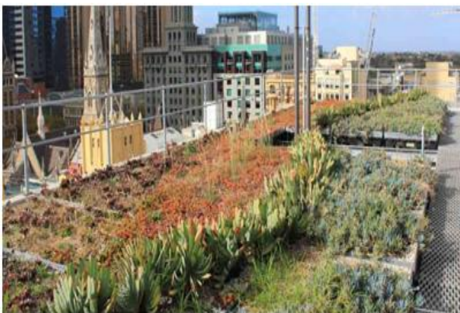
Figure 1.7: Sustainable roof at Council House 2, Little Collins Street, Melbourne
