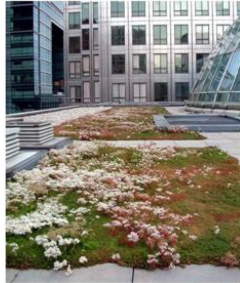
Figure 2.2: The School of Art and Design in Singapore is an example of a simple-intensive green roof
