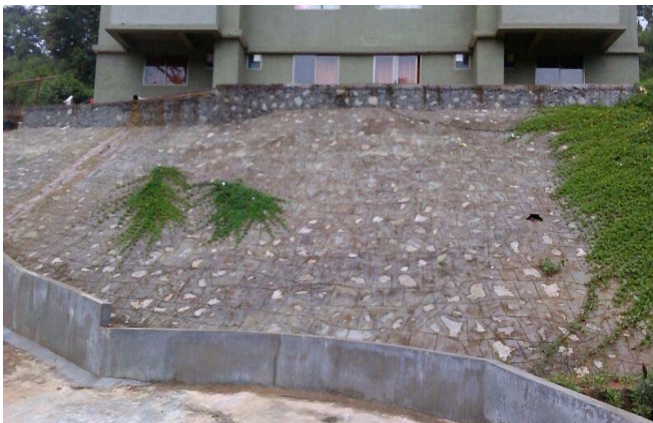
Figure 6: stones and cement is used at slopping area near the building to prevent land sliding and giving strength to the foundation of the building.
