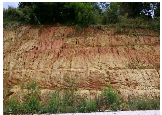
Figure 3: stepladder cutting of hill while making road
