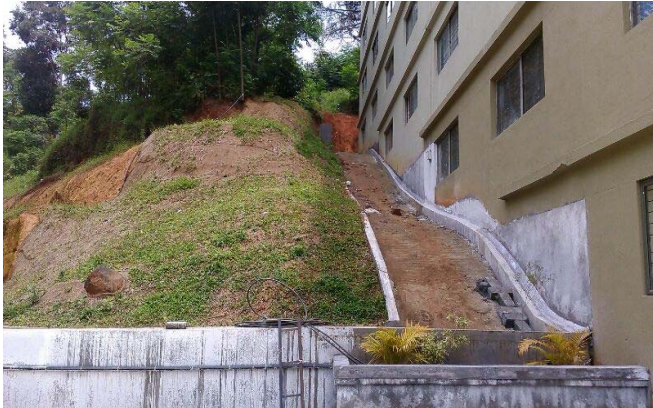
Figure 5: putting a concrete around the constructed building and plantation at the slopping area to give strength to the soil.
