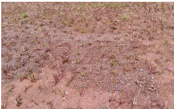
Figure 7: plantation is done at slopping area by using biodegradable mesh, which gives strength to the plants and its roots.
