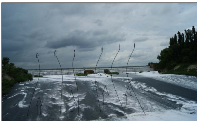
Figure 3: Represents the ground level air turbulence generates the rapid bioaerosols emission from outlet weir
