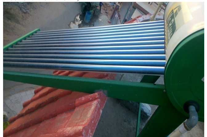
Figure 1: Solar Water Heater Using Vacuum Tubes
