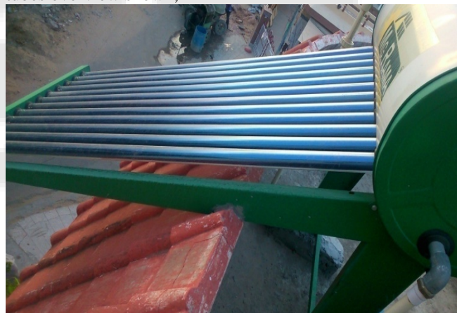
Figure 1: Solar Water Heater Using Vacuum Tubes
