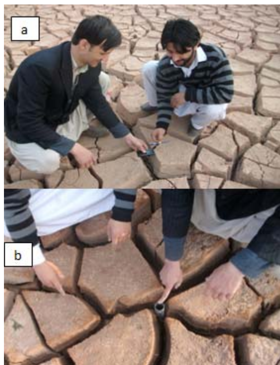
Figure 02: a width of the crack, b depth of the crack Crack pattern of expansive soil
