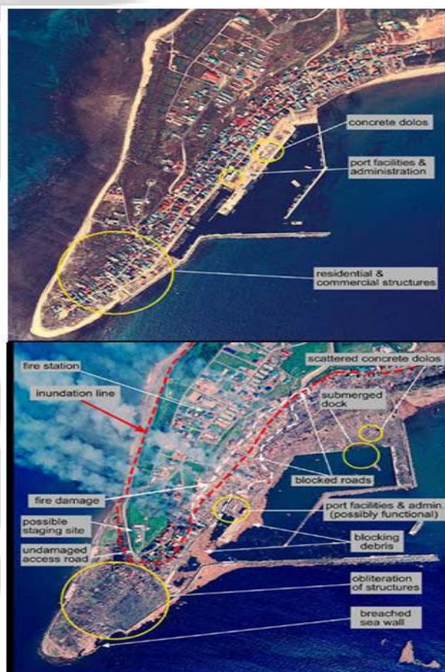
Figure 4: Aerial photo of before and after tsunami hit an area [9]
