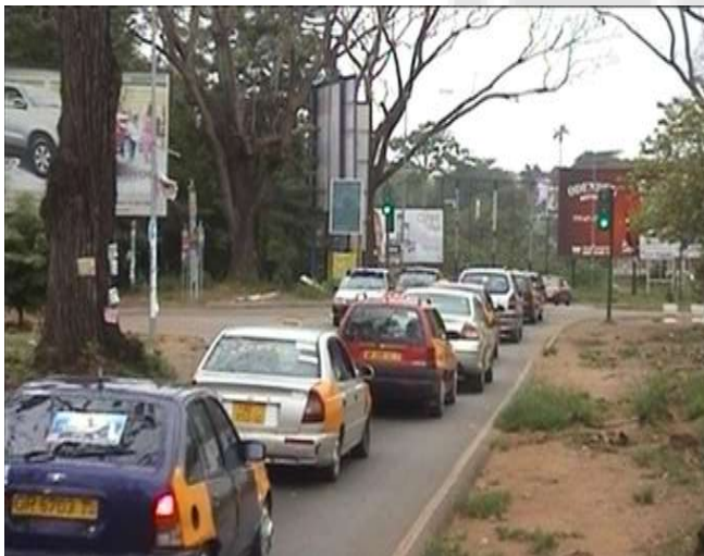
Figure 2: The Pine Avenue Signalized Intersection (none/low roadside friction)
