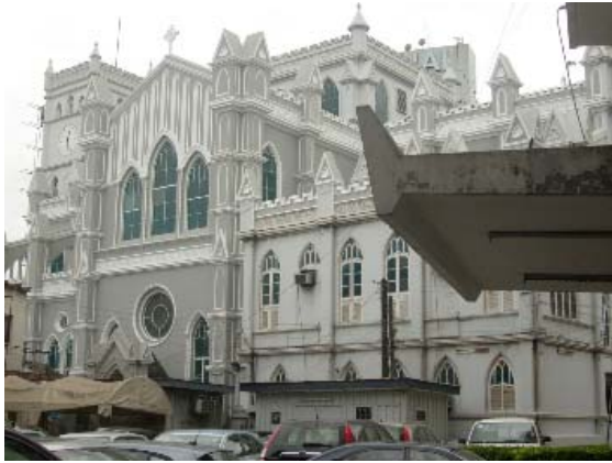
Plates 4.1.1: External views of The Cathedral Church of Christ, No. 29 Marina, Lagos (1925-1946) field study picture in March 2008
