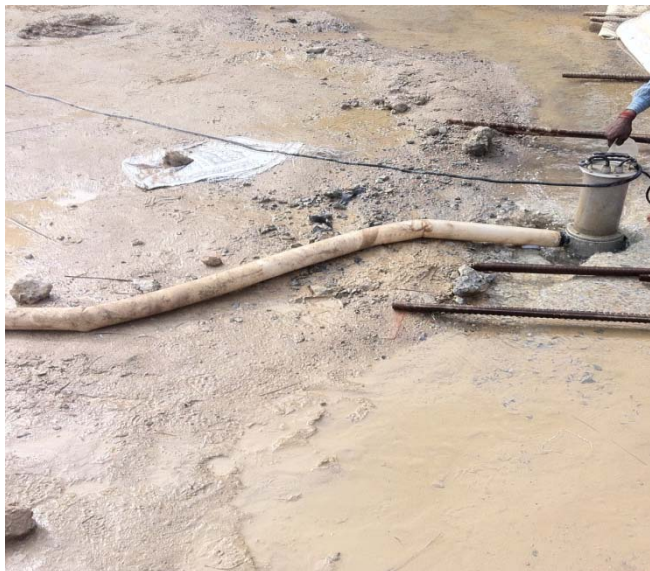
Figure 1: Deep Well Pump Dewatering System Used For Dewatering Excavated Area
