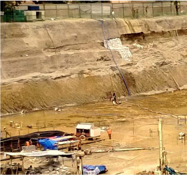
Figure 4: Stabilization of Slopes By Soil Nailing And Shotcreting.
