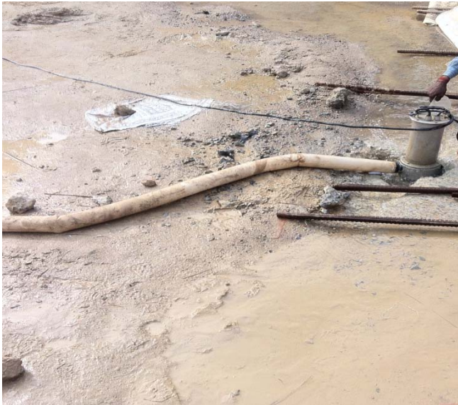
Figure 1: Deep Well Pump Dewatering System Used For Dewatering Excavated Area
