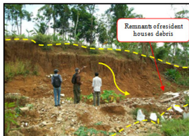
Figure 9: Remnants of resident houses debris that have been affected by landslide (yellow arrow represent direction of landslide)
