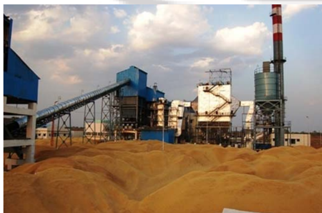
Figure 4: 10 MW Biomass Power Project, Gadchiroli Dist. (Maharastra)
