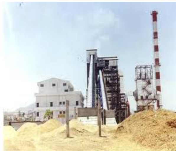
Figure 5: 18 MW Biomass power project in Tamilnadu
