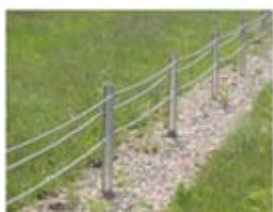
Low-tension cable barrier
