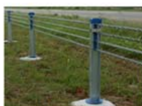
High-tension cable barrier
