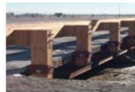
Timber Bridge Rail
