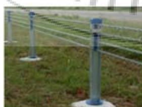
High-tension cable barrier
