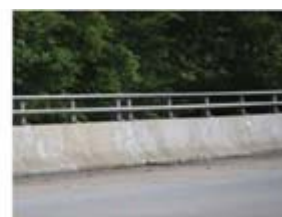
Vertical Concrete Parapet
