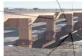
Timber Bridge Rail
