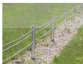
Low-tension cable barrier
