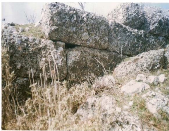
Figure 7: Tract wall on the southeast side
