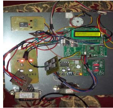
Figure 2: Transmitter Section inbuilt in the vehicle
