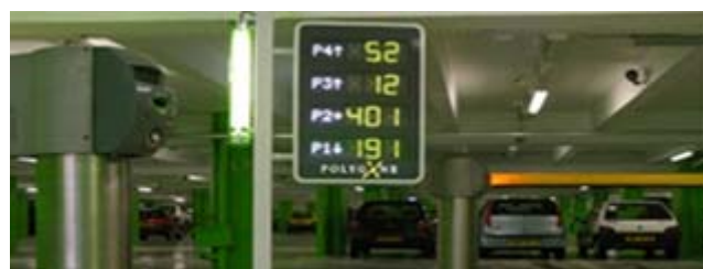
Figure 1: A typical Parking Guidance Information System
