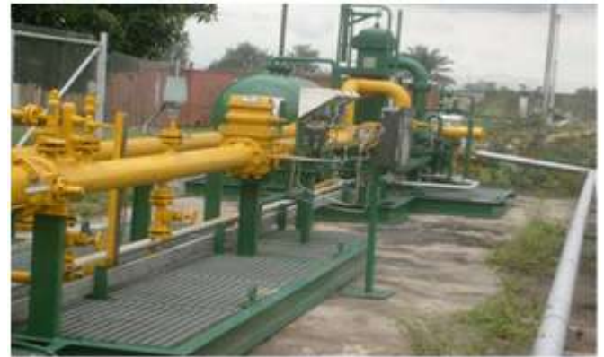
Figure 3: Natural Gas (fuel) Lines
