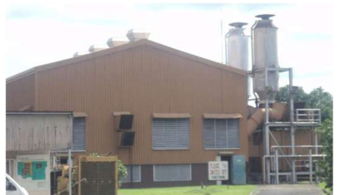
Figure 1: The Central Power Plant (Shell, Edjeba)
