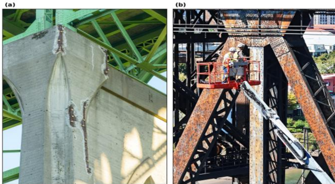
Figure 2: Field deterioration and access challenges in aging bridges: (a) concrete spalling on pier columns; and (b) close-range inspection of corrosion-prone steel members using an aerial work platform.
