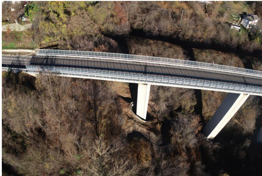
Figure 4: Real bridge inspection view acquired from an unmanned aerial vehicle, with field survey targets and antennas supporting geometric control
