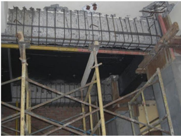
Figure 3: Jacketing of Beam on site
