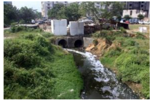
Figure 6: Sewage and untreated wastewater flowing into Makarba Lake
