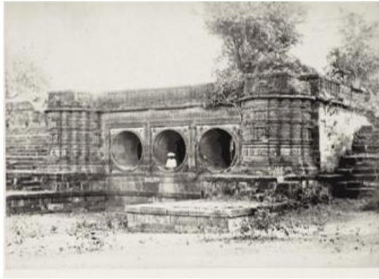
Figure 4: Howz-i- Kootub, Kankaria Tank- The Supply-Sluice
