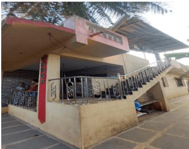
Figure 5: New house of RCC construction, covered with sloping steel profile roof for protection from rains and subsequent leakages. (Source: Authors)
