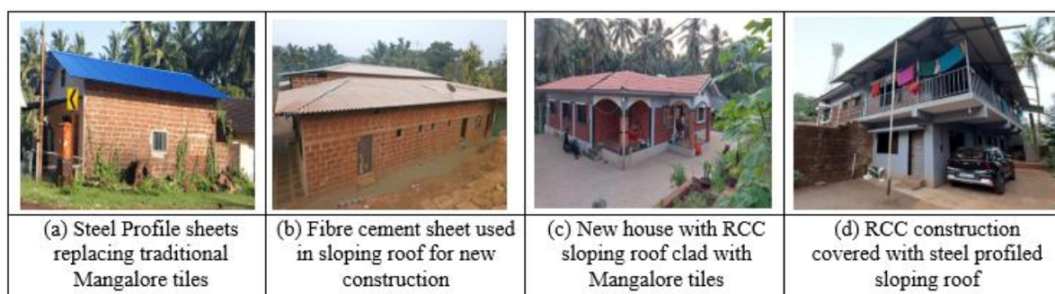
Figure 4: Progressive roofing interface
