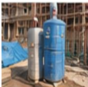
Drinking Water Point
