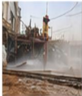
Water Sprinkling (Dust Control)
