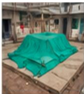
Material Covered (Stockyard)
