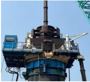
Figure: RCD/BHA dismantling from Pile
