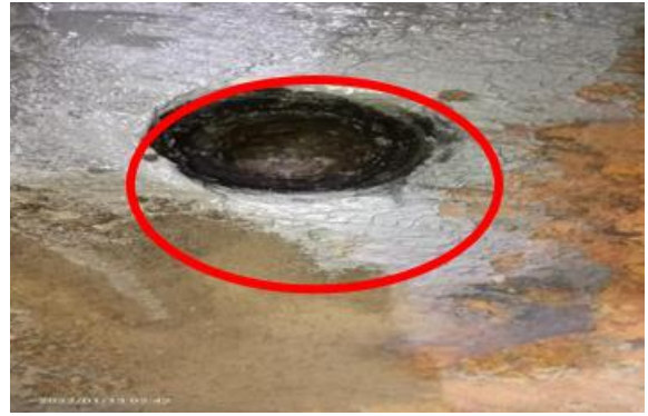
Figure: Outlet pipeline after slush removal
