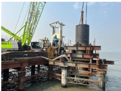
Figure: Plug concrete between outer & inner liner to counter the wave impact on liner.
