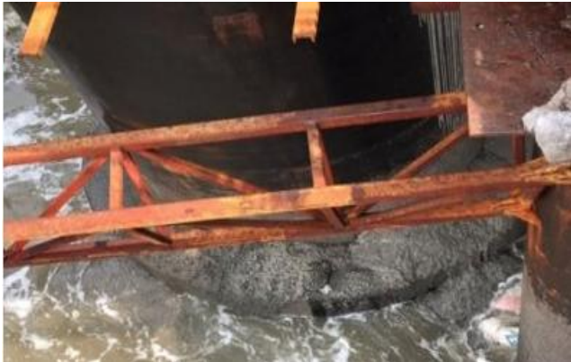
Figure: Plug concrete between outer & inner liner to counter the wave impact on liner.
