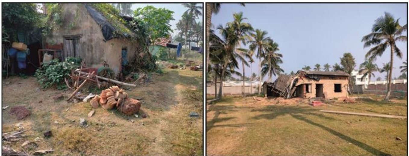
Figure 4: The figure shows field photographs of cyclone-induced damage to local houses in coastal areas. (A) Partially damaged mud house with scattered household items and overgrown vegetation indicating neglect. (B) Severely damaged brick house with collapsed roof structure, highlighting structural vulnerability to extreme weather events.
