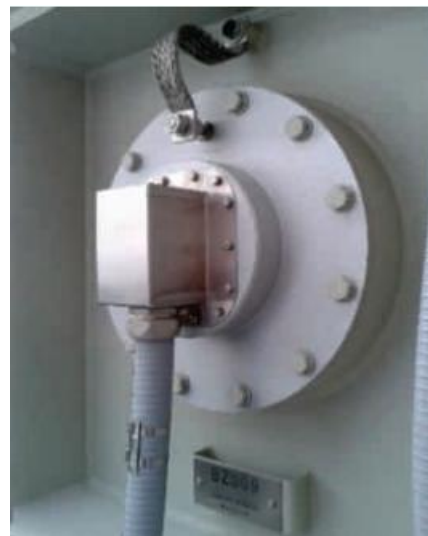
Figure 6: UHF disk sensor on the transformer tank
